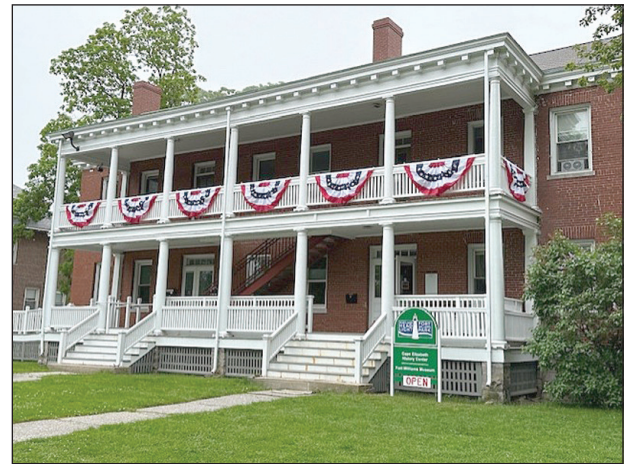
The former Bachelor Officer Quarters at Fort Williams Park is just a short walk from Portland Head Light.
