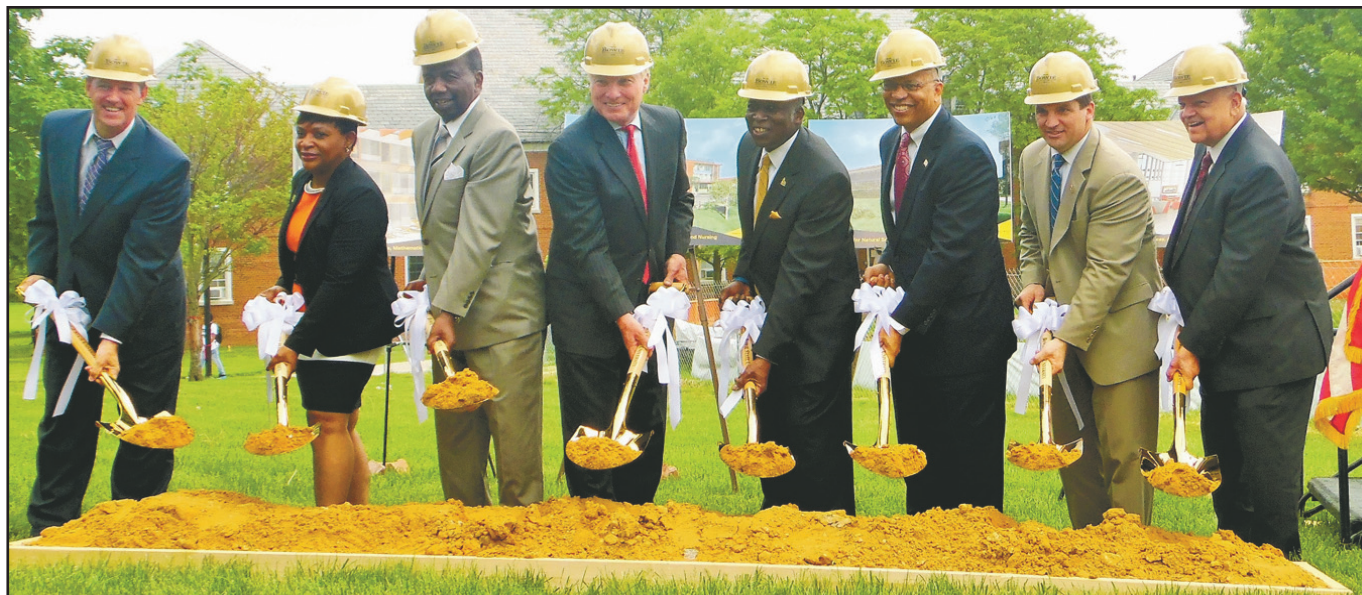
Maryland Lt. Governor Boyd Rutherford joined other state elected officials on Bowie State's campus to mark the groundbreaking for the Center for Natural Sciences. (Left to right) David Tacchetti, vice president of Clark Construction Group; Maryland Delegate Adrienne Jones; Maryland Senator Ulysses Currie; Comptroller Peter Franchot; Bowie State President Mickey L. Burnim; Lt. Gov. Boyd Rutherford; State Senator Douglas J.J. Peters; and Maryland Delegate James Proctor Jr.
