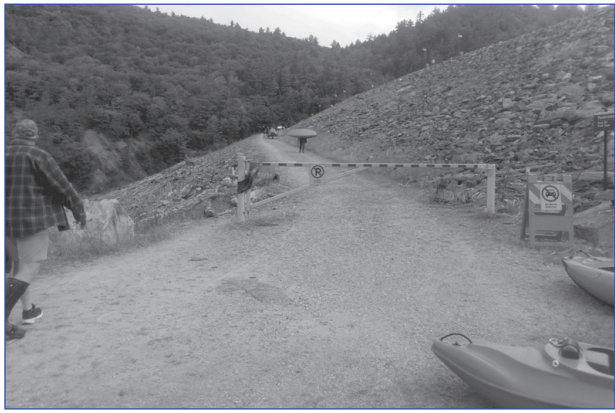
A kayaker begins the climb up Ball Mountain Dam
