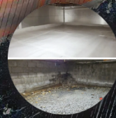
Crawl space Structural Repairs
