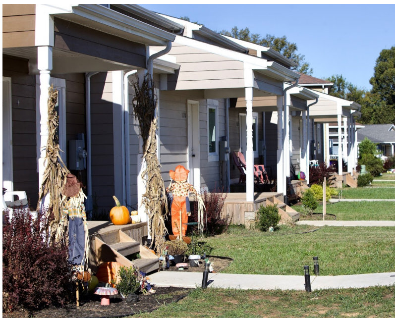
▲ Several of the team's completed projects
