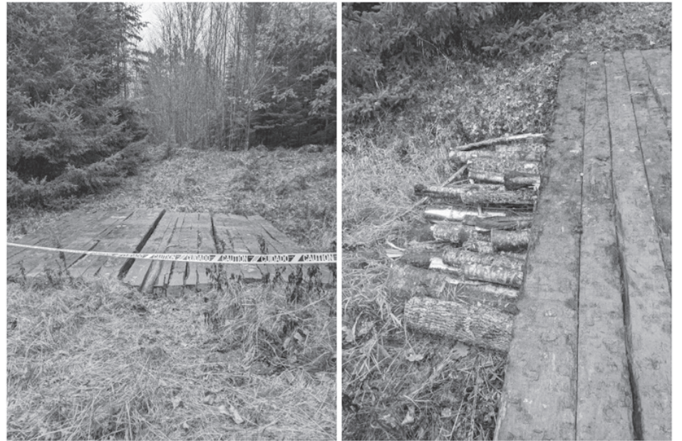
Crossing constructed to access drilling location. Photo credit: Jill Howell, Upstream Watch
