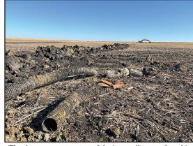
The three common types of drainage tile were found in one area, representing the major efforts to drain this shallow lake since the 1920s. Plastic, clay, and cement tile can be seen along the trench they were removed from. Photo by Jake Chronister, Ducks Unlimited.
