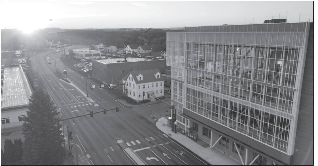
Vertical Harvest facility in downtown Westbrook.
