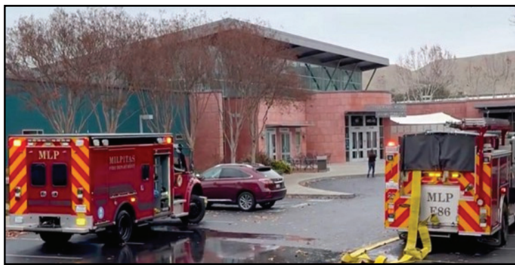
The Humane Society of Silicon Valley in Milpitas is recovering from a fire that broke out Dec. 16 and destroyed half of the building.
