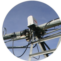
Tower Box Conversion
