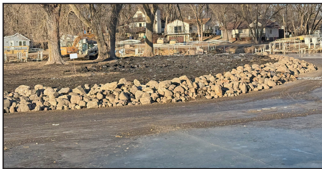
(photo by Steve Weisman) Rock barrier designed to protect the island from future erosion.
