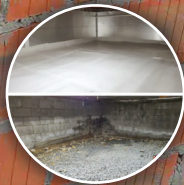
Crawlspace Encapsulation
