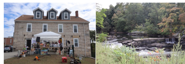
Site of still standing Charles Lee Mill Store in Willimantic and remains of millworks.
