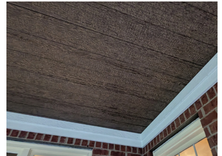
Porch Ceiling: LP SmartSide ExpertFinish® Nickel Gap Siding in Weathered Walnut Cedar Texture
