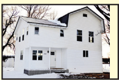
Chittenango $105,000 Remodel in progress. Finished this home the way you want. Chittenango Schools. Peter Denney 247-1910 (D)
