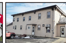
Vernon $124,000 Loads of potential prime location, brand new furnace, 3BR Apt. priced right. Michael Shue 345-3311 (C)
