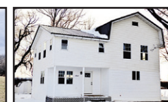
Chittenango $105,000 Remodel in progress. Finish this home the way you want. Chittenango Schools. Peter Denney 247-1910 (D)
