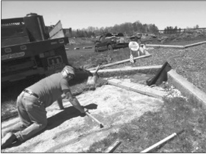
Keith G. Millett, owner of K. G. Millett Masonry of Turner, prepares the important leveling and grading before installing the pavers on the walkway to the Gold Star Mothers Monument.
