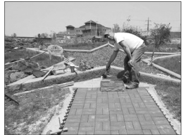
Working on the pavers.
