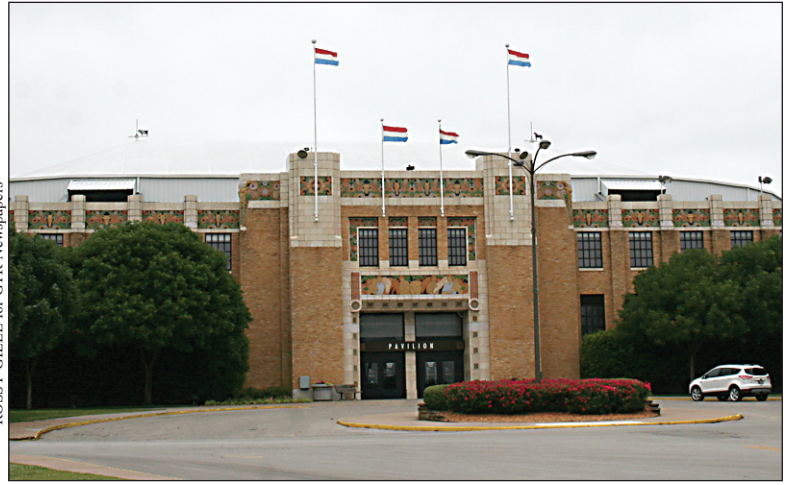
NOTEWORTHY ART DECO: Expo Square Pavilion is one of Tulsa's noteworthy Art Deco buildings. It was built in 1932 and designed by architect Leland L. Shumway. The Pavilion had an original seating capacity of 10,000 people, which, at the time that it was built, made it the largest auditorium in Tulsa. A floating roof system supported by long span trusses, creating a dome, allows the interior to be column free.
