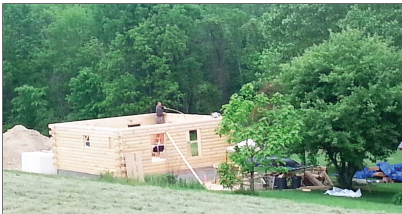
Allegany Log Home from Houghton, NY going up for staff housing.
