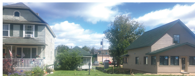
Basement flooding in home (center) blamed on new construction (right).
