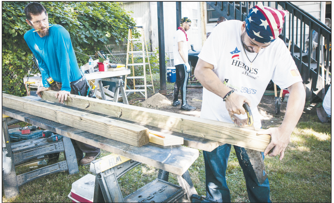
Sears Heroes at Home teamed with nonprofit Rebuilding Together Baltimore as a team of more than 20 Sears volunteers helped repair and renovate U.S. Army and Reserves veteran Charles Faison’s home of 52 years. In addition to the stairs, repairs included fixing damaged ceilings, roof patching, a new Kenmore stove, accessibility upgrades and more.
