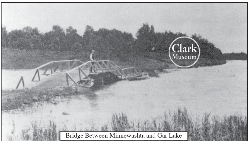
Bridge Between Minnewashta and Gar Lake
