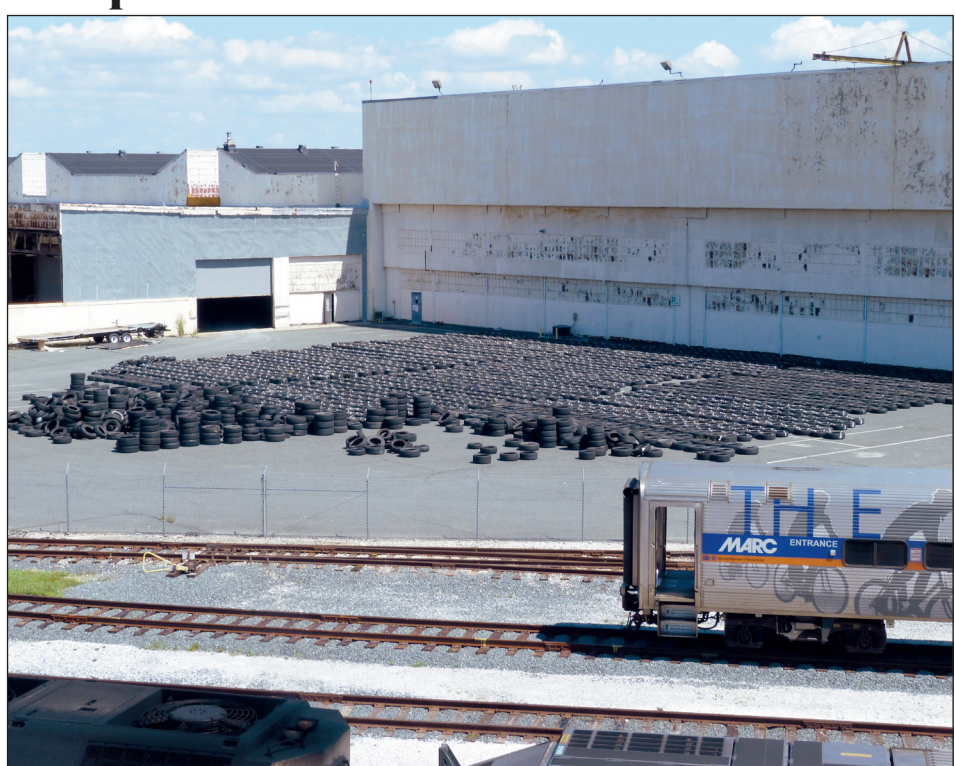
The mass of tires, visible here from atop MD-43, is outside the main building at the Depot, between the building and the state property used by the Maryland Transit Authority's MARC train.
