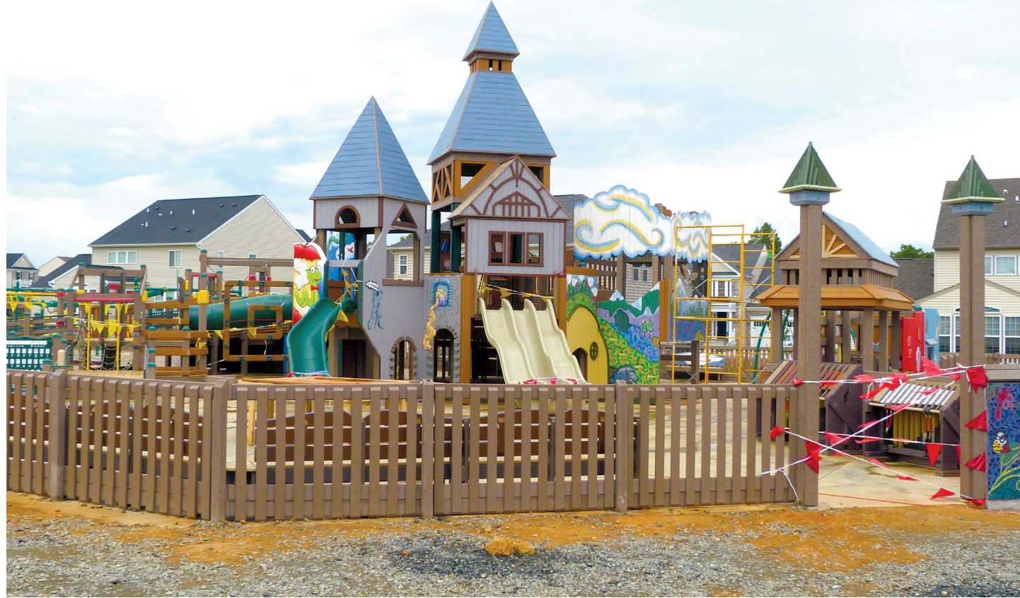
The completed Angel Park equipment stood Monday awaiting only its rubberized flooring and for every child visitor to be able to climb to the top of the castle.
