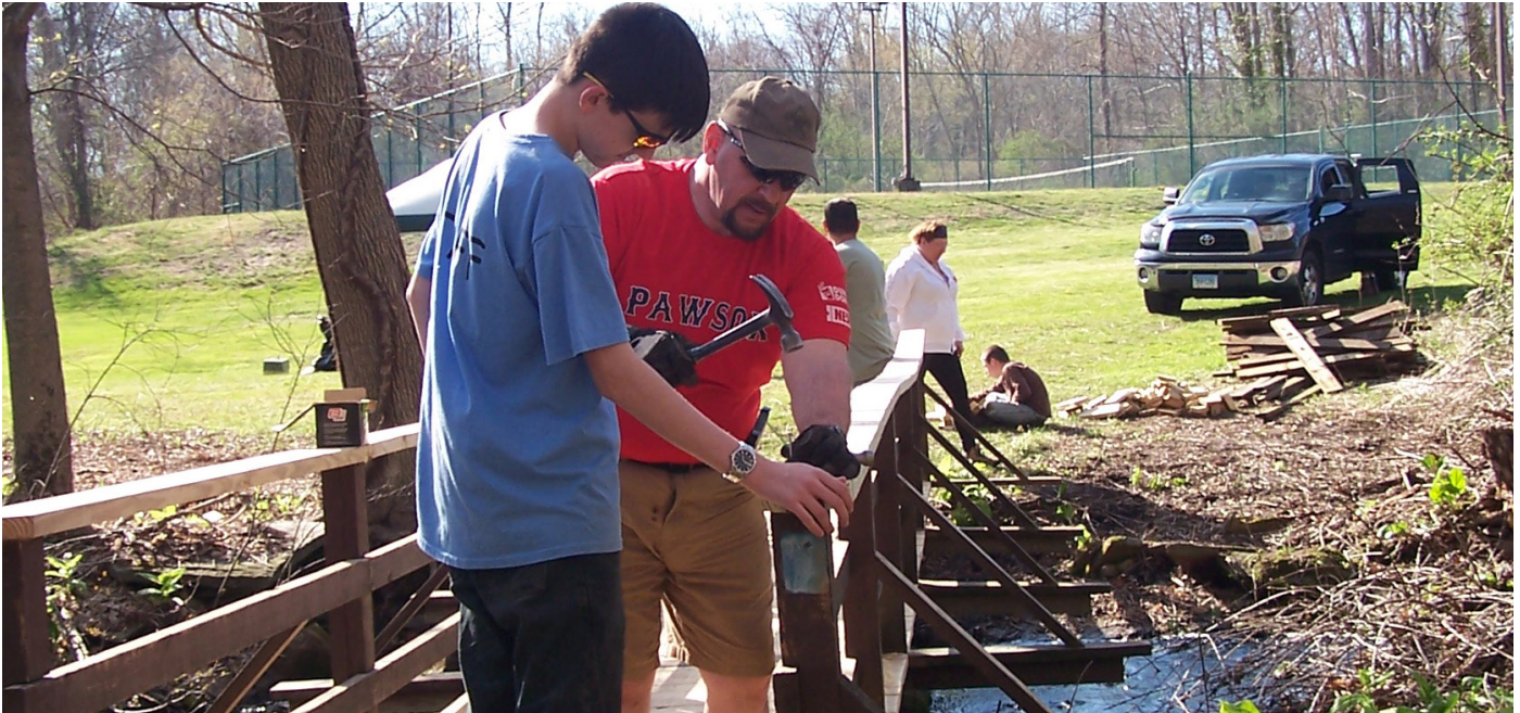
Life Scout and Eagle Scout Candidate Richard L. LaBonte, Jr. (left), holds a board as his Scoutmaster, Peter A. Lombardo, of Putnam, drives a nail, as part of the construction of the new footbridge over Creamery Brook in Brooklyn. Vikki LaBonte photo
