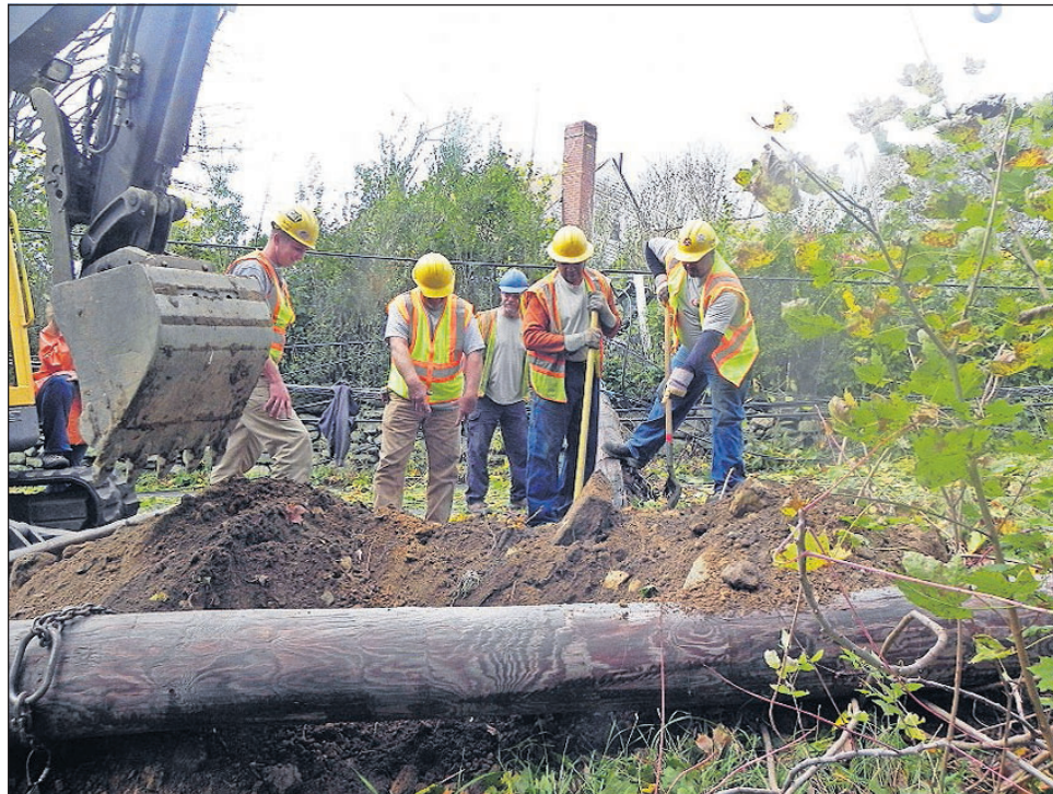
Norwich Public Utilities makes repairs after Tropical Storm Sandy.
