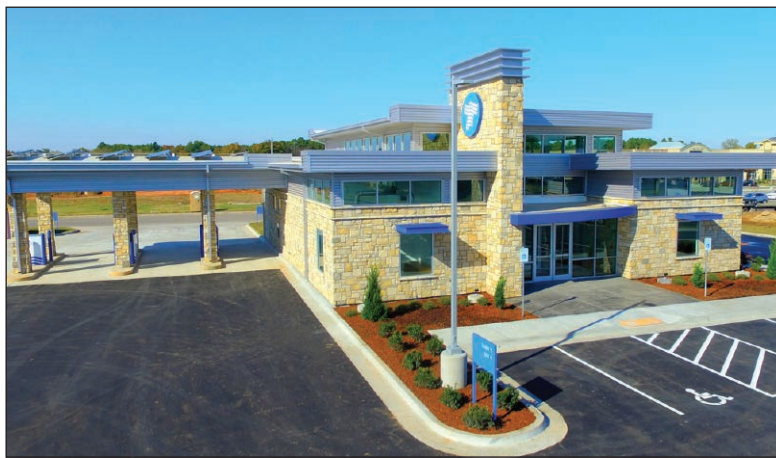
STATE OF THE ART FACILITY: The new Tulsa Federal Credit Union location will offer one of the most up-to-date financial facilities anywhere.
