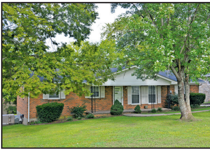
143 Circle Dr, Fayetteville -is move in ready! This 1,144 SF Brick Ranch House features 3 BR, 1.5 BA, living room, kitchen/dining combo, 1 car garage/utility. Other features include new windows, detached carport and utility building. Located in a very nice, well-kept neighborhood. $85,000
