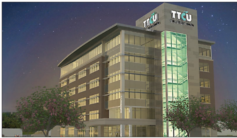
IMPRESSIVE BUILDING: TTCU's corporate headquarters has an expected completion date of late 2016. The new facility will be located next to TTCU's Southeast branch location near 81st Street and Highway 169.
