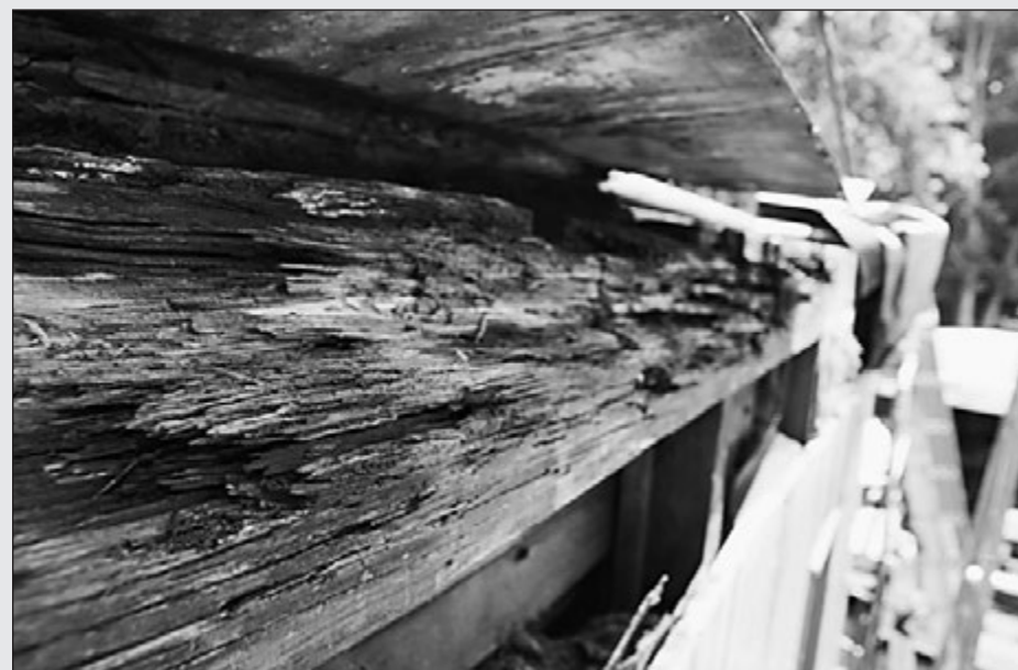
This is what the cupola looked like when work began.
