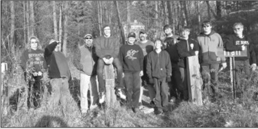
Led by Dylan Latham of Boy Scout Troop 007, volunteers removed trash, replaced bollards, filled in holes, and built an arch.
