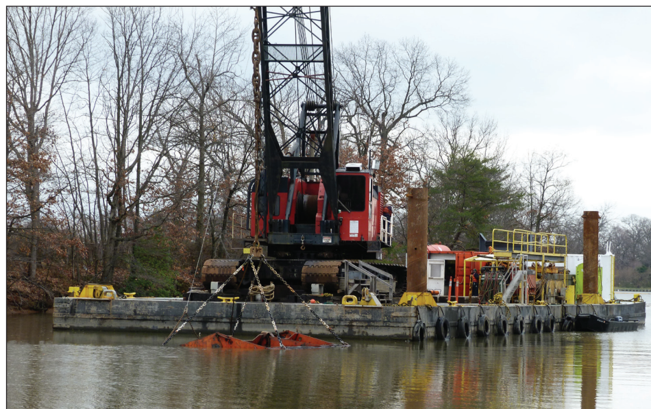
One of the barges as it dredges up the work area in Cowpen Creek.
