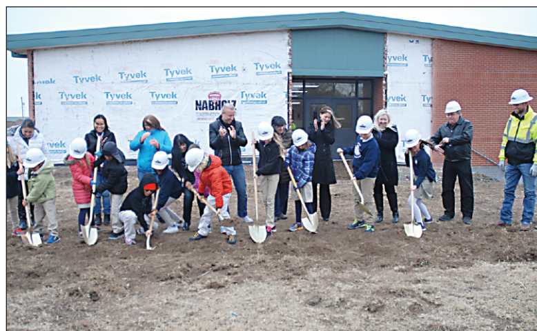
INCREASING SAFETY: On Dec. 16, Zarrow International School and Nabholz construction broke ground on a 7,000-square-foot building that will include six classrooms for grades fourth and fifth and also serve as a safe room. A new bus loop will be added on the east side of the facility to increase traffic flow. The project is expected to be completed in October.
