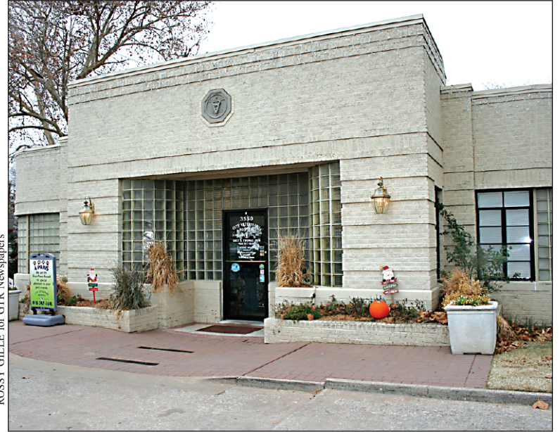
CITY VETERINARY HOSPITAL: At 3550 S. Peoria Ave., it was designed by Joseph R. Koberling in 1942 and has operated continuously as a veterinary clinic.
