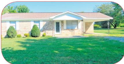
390 Limestone Rd. - Sweet 3 BR recently updated home in Elora. 3 BR, 1 BA. New ceiling fans, new carpet, new vinyl, new laminate, new pantry and updated kitchen cabinets. New paint. 1,280 sq. ft. full brick home. MLS#1764764 $67,000
