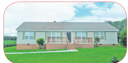
528 Limestone Rd. - Well maintained manufactured home on permanent foundation w/ large rooms, crown molding, recessed lights and wood burning fireplace. Beautiful view of surrounding fields w/ room to garden and large yard. 3 BR, 2 BA home. Storage building. MLS#1757064 $89,900
