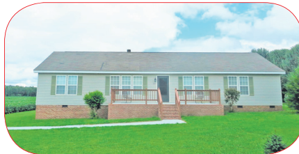
528 Limestone Rd. - Well maintained manufactured home on permanent foundation w/ large rooms, crown molding, recessed lights and wood burning fireplace. Beautiful view of surrounding fields w/ room to garden and large yard. 3 BR, 2 BA home. Storage building. MLS#1757064 $89,900
