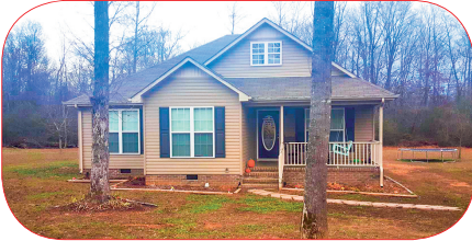
8 Timber Edge Rd. - Very nice home on over an acre. Home has vaulted ceiling in the living room, island in the kitchen, split floor plan, laminate floors, nice covered porch and a deck. All info TBV by the buyer. MLS#1789289 $108,000
