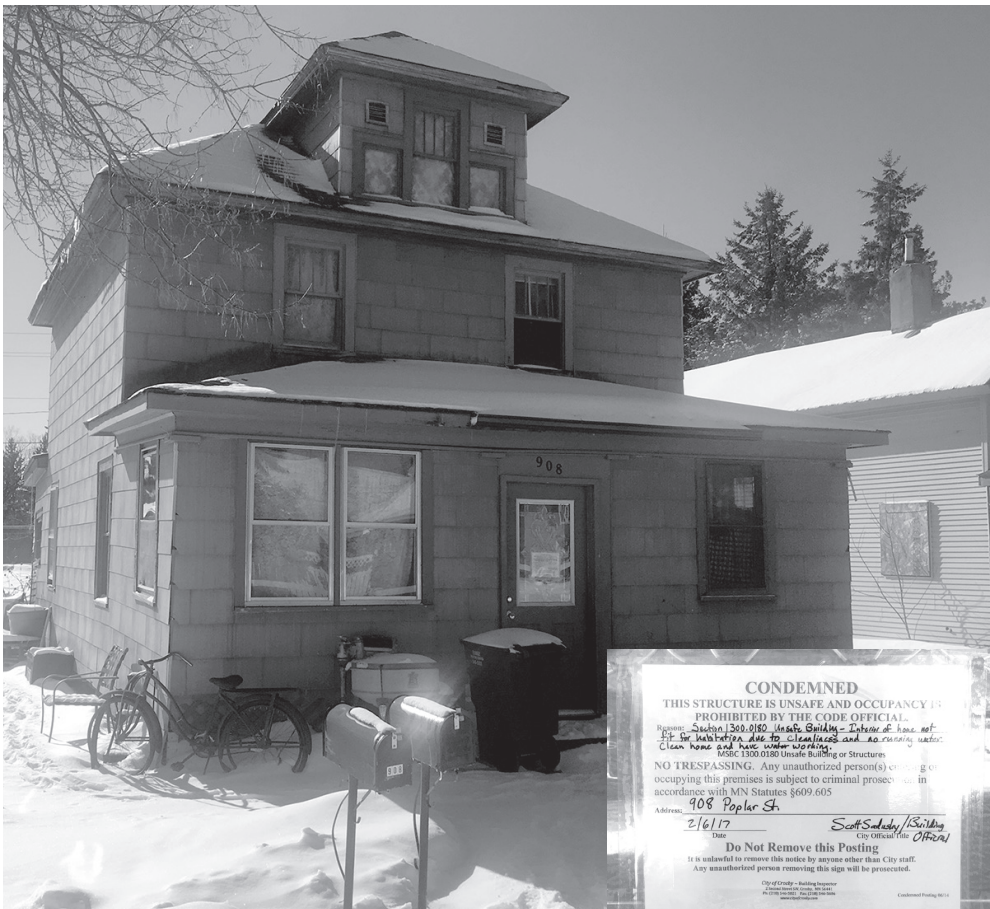
The City of Crosby condemned a house at 908 Poplar Street in Crosby on Monday, February 6. It was determined that the interior of the home was not fit for habitation, due to cleanliness and no running water. Crosby and Deewood police officers, with the assistance of the Humane Society, removed 27 cats from the home.
