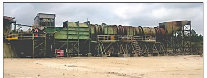
90 Ton/Hr. Complete Chip Mill
