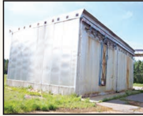
American Wood Dryers Kiln
