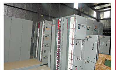
Truck Loads of Electrical
