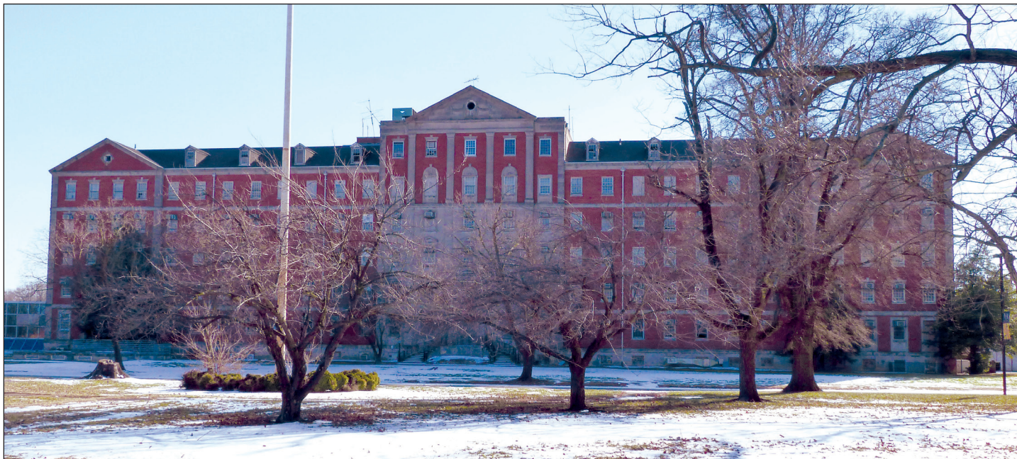
The VA hospital building was one of two buildings on the site specifically named as needing to be secured because of open elevator shafts inside them. Signage must also be installed by March 3 warning trespassers of the danger. File photo.
