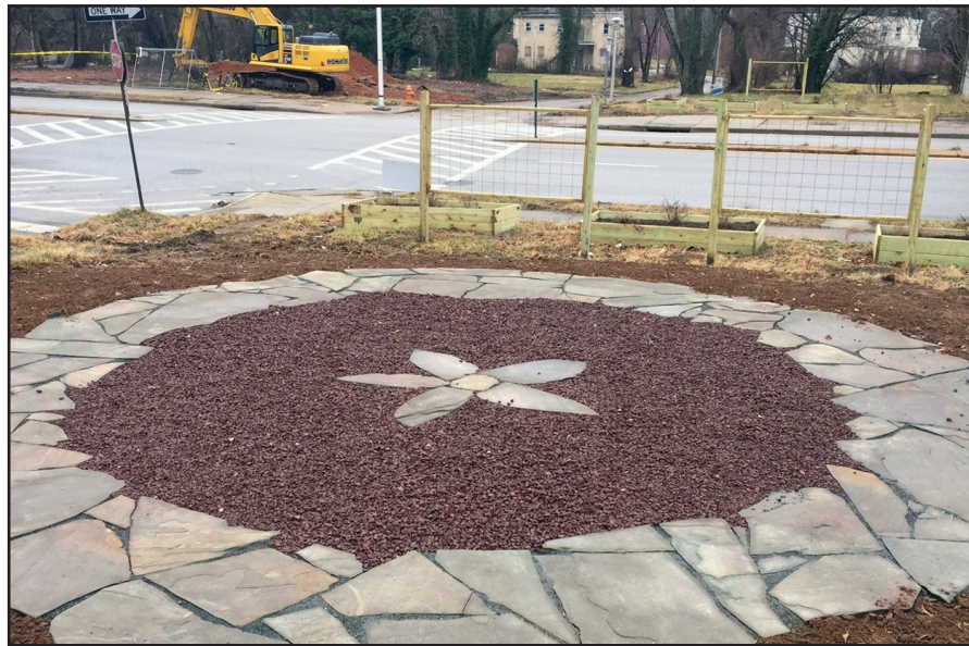
A new gathering space at 4701 Park Heights Avenue for children waiting at bus stop after school. Courtesy Photos/Civic Works
