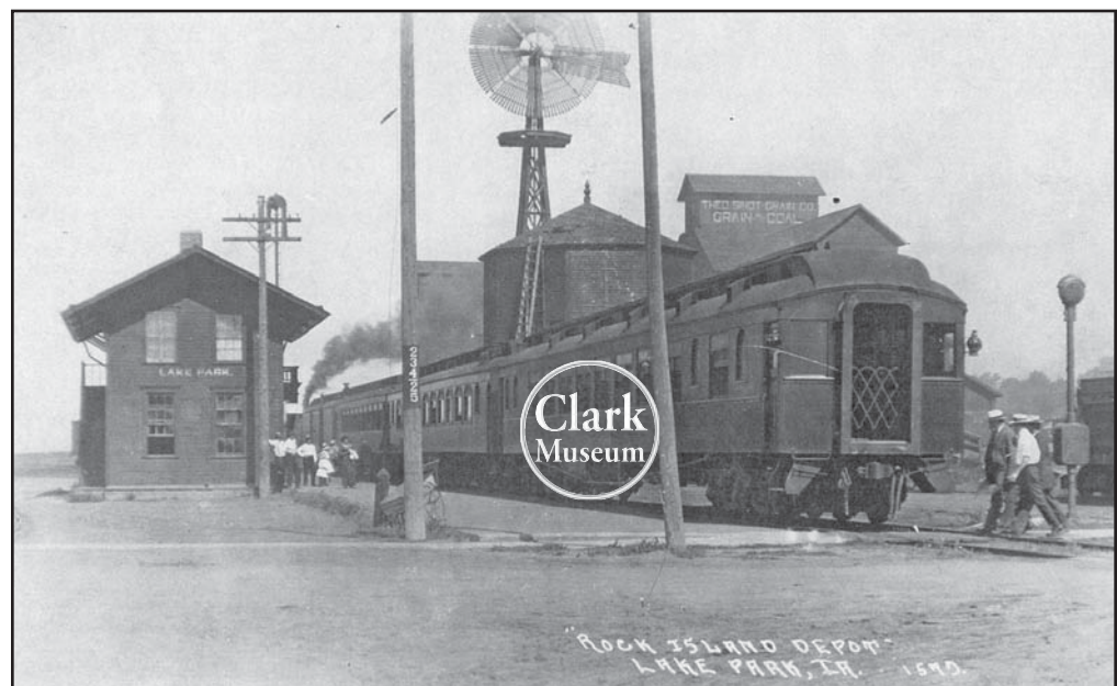
Rock Island Depot, Lake Park, Iowa • Early 1900
