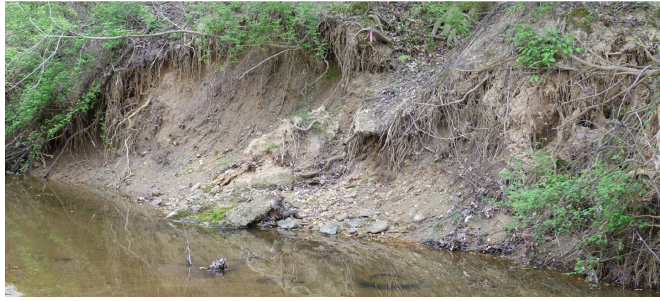
Stream bank erosion, as seen here along Honeygo Run in White Marsh, is the main cause of sediment pollution in the Bird River.
