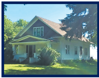
911 ALBANY AVE NE $275,000
