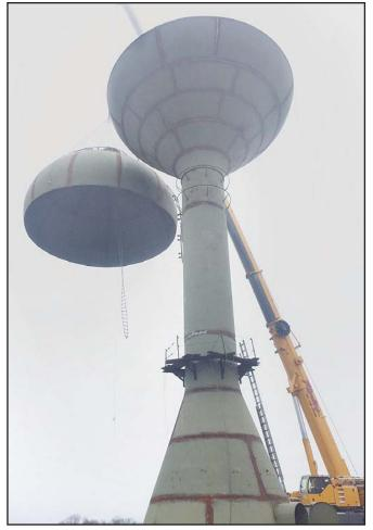
WAHPETON WATER TOWER COMPLETED - After more than a week of weather-related delays in hanging the cap of the tank on the new Wahpeton water tower at the High Point site on Iowa Highway 86, the job was finally completed in foggy conditions, less than two hours, just before 8:00am, Tuesday, April 25, 2017. The 200,000-gallon, \$928,000 project quadruples the system's capacity, and should be completed in time for peak use of the water system in July. Photo by Lars Dilling, Maguire Iron Services
