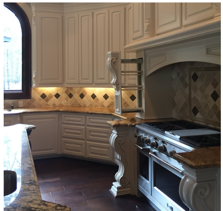
Oversized corbels in areas of traffic can be a nuisance.
