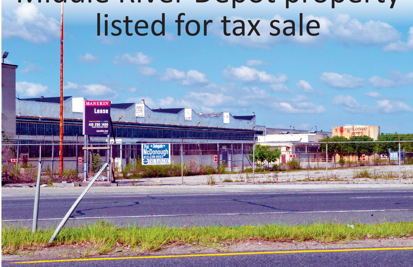
The main building on the depot property has been largely unused since the current owner purchased it in 2007, despite a major redevelopment plan for the entire site on file with Baltimore County. Photo by Devin Crum.
