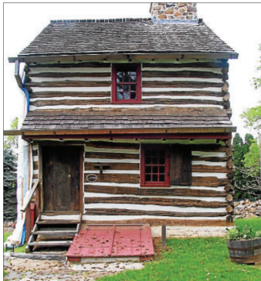
The Southery Log House.
