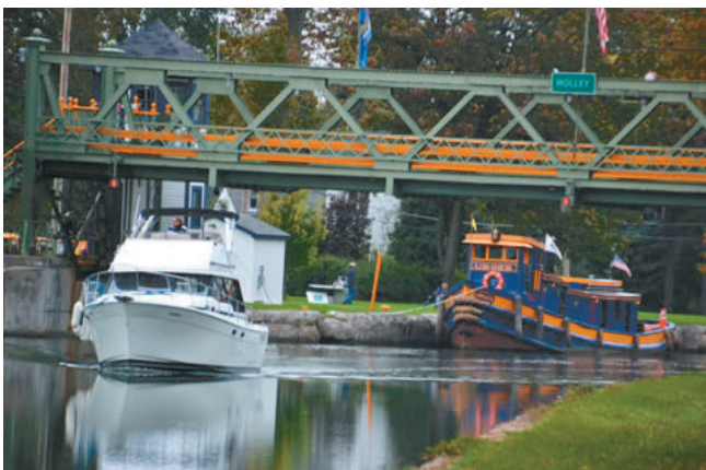
The lift bridge in Holley goes up to make room for a modern boat. The historic Urger, a tugboat from 1901, is pictured in back.
