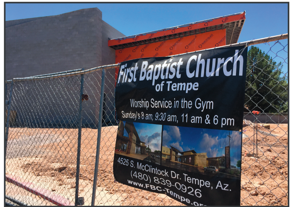
The new sanctuary at First Baptist Church of Tempe is beginning to take shape as the year-long, $8 million project unfolds on the church campus near McClintock Drive and U.S. 60.
