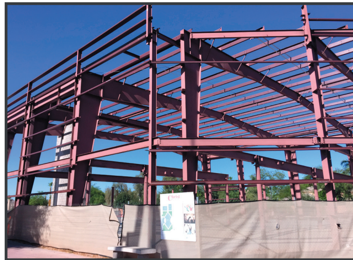
Christ Life Church in Tempe, a non-denominational congregation, is in the midst of a major construction project.
