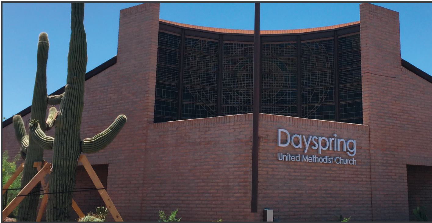
Dayspring United Methodist Church in Tempe has updated its Sunday school and preschool classrooms as well as upgraded landscaping on the property. A new digital sign and repaved parking lot are also part of the refurbishing.
