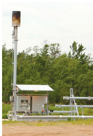
Crow Wing County Landfill gas flare is utilized to combust the landfill gas collected within the landfill.
