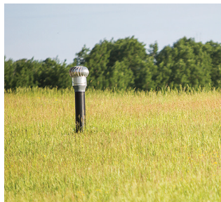
Landfill technology changes: here is a methane gas vent pipe from an inactive gas well in the old landfill that was closed in 1992. The current landfill has an active gas system that gathers all the gas to be sent to the gas flare (pictured at right.)
