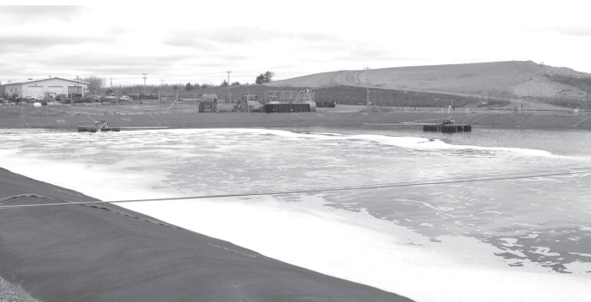
A closer view of one of the on-site water leachate treatment ponds, Leachate Pond 4. The pond has a capacity of 2.4 million gallons and is aerated for treatment. The onsite system protects water quality and saves taxpayers about $500,000 a year.
